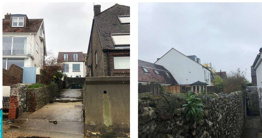
View from Harbour and west (side) elevation
