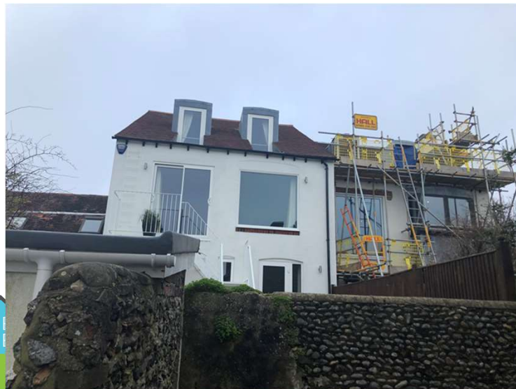
View from South of Existing Rear Elevation
